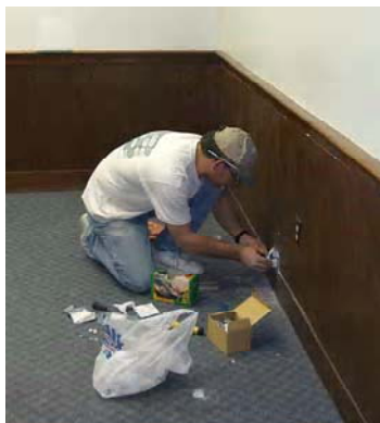
Steve Roszhart from Aldersgate helps install new phone and computer outlets.
